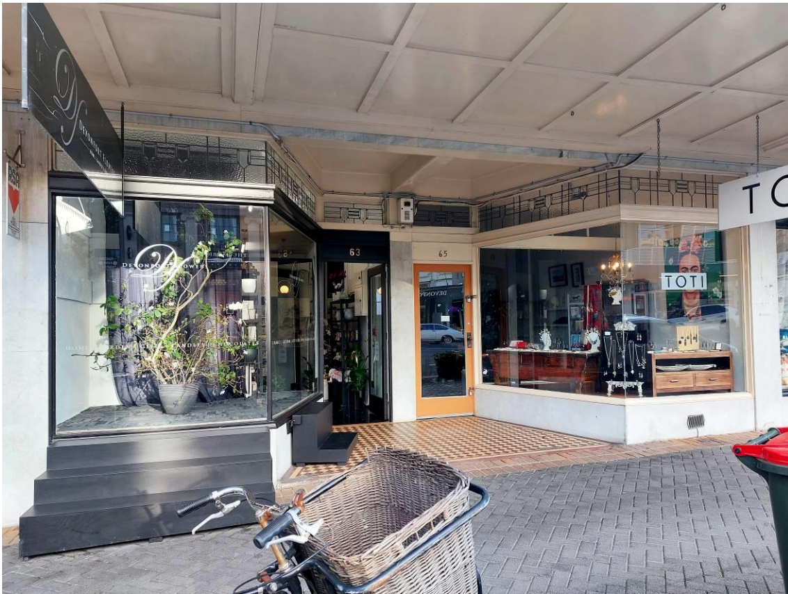
Figure 38 Devonian Building - unmodified ground floor shopfronts
