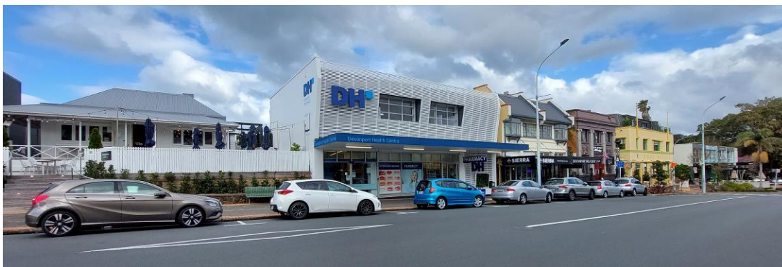
Figure 26 Typical view on eastern side of Victoria Road
