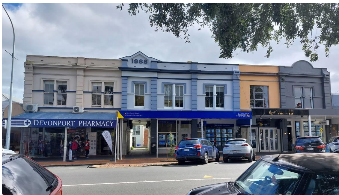
Figure 23 Typical view on western side of Victoria Road
