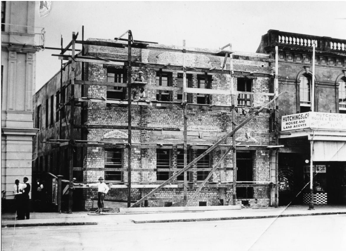
Figure 8 Devonport Post Office being remodelled for the new Borough Council Chambers 1939
